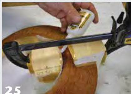
25 Custom clamping blocks, aka a compression mold, help to apply localized pressure, as a stubborn section of veneer is re-glued.
