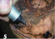
the area of the first epoxy pour. A rotary tool is used to widen some cracks to facilitate a more thorough flow of epoxy.
