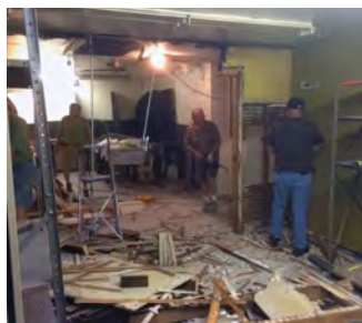
The DAW crew knee-deep in demolition, knocking down walls and moving electrical and plumbing, to make smaller units into a larger, more functional space.
