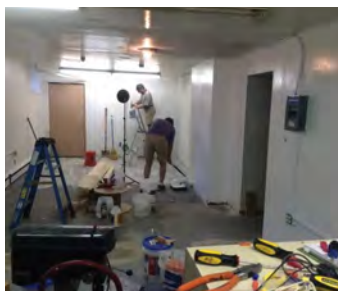
Reconstruction involved updating and adding light fixtures, drywall, and paint, as well as filling, leveling, and sealing the floor.
