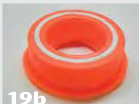
19b With the protrusion cut away, the coupling can be removed.
